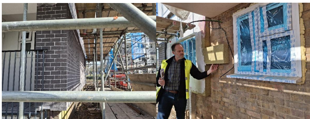
Figure 14. SHDF Wave 2.1 retrofitting works.
